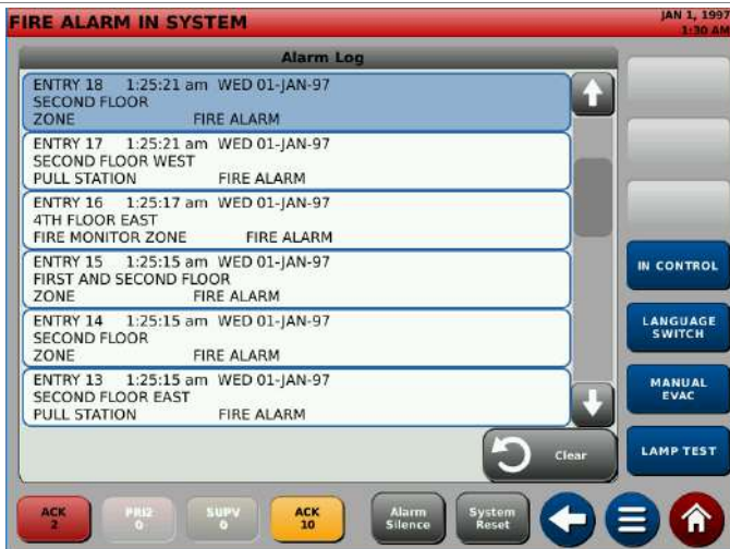
Figure 14: Alarm History Log
